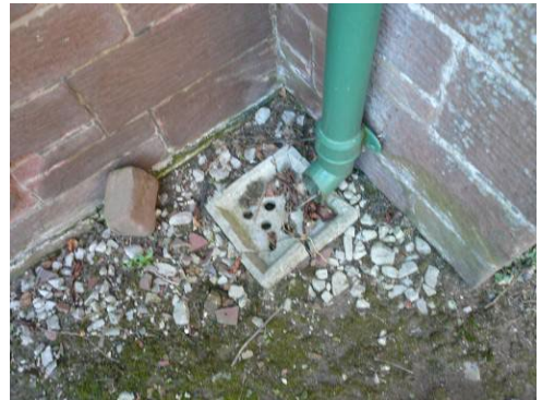
Cracked gully
