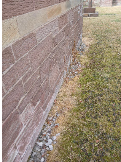
Vegetation in French drain gravel.
