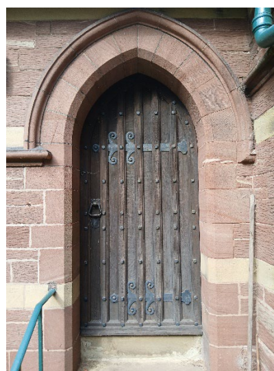
Vestry door (external face)
